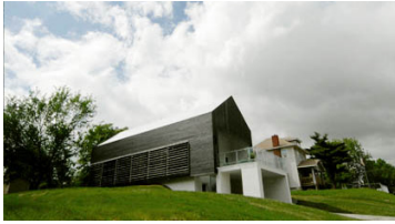
2010 32 S 16th Street, Kansas City, KS LEED Platinum Certification , U.S. Green Building Council, 2010
